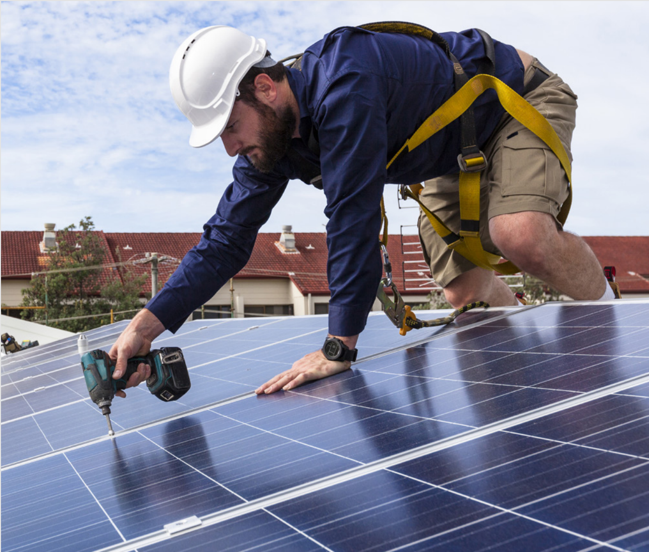
Solar panel technician with drill installing solar panels on roof @zstock/shutterstock
